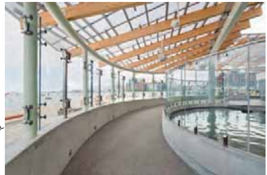
Glass is the dominant design feature of a recently completed exhibit at the New England Aquarium.
