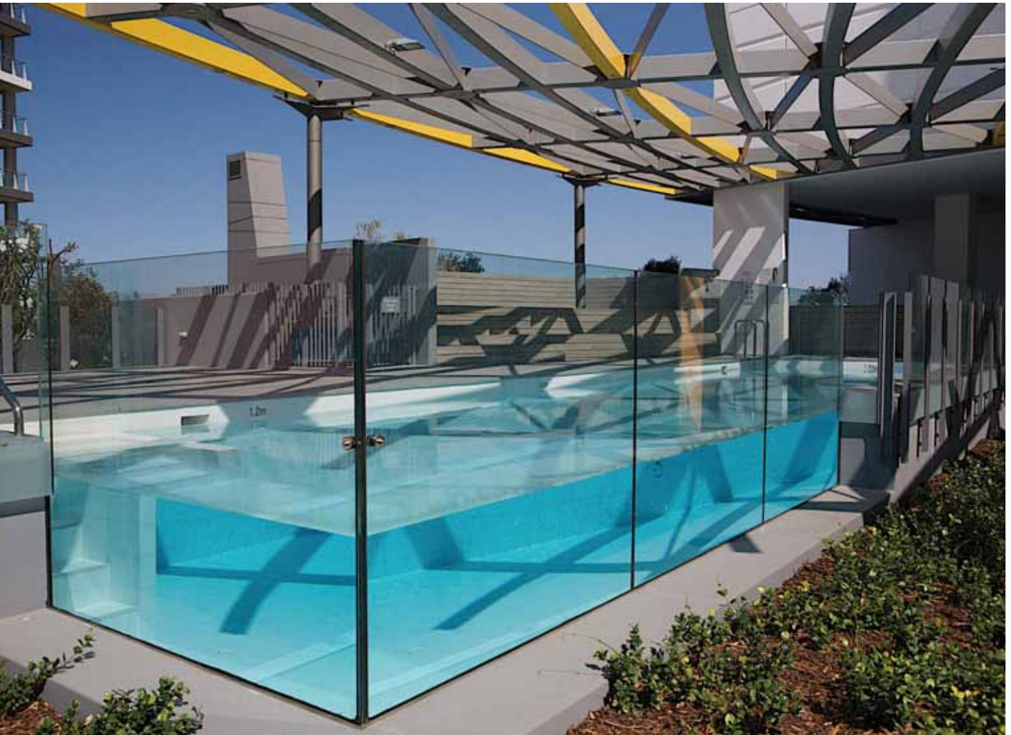
Glass pool walls, such as the one installed at the Tower 4 Burswood Complex in Western Australia, are becoming popular design features.
